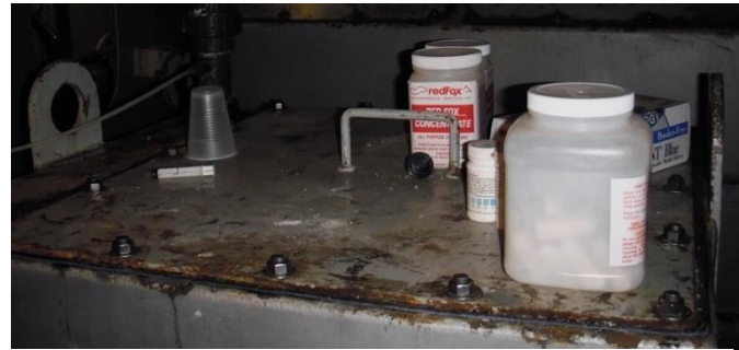
Figure 3 Tank Top With Bolts to Allow Opening
