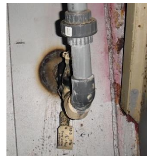
Figure 2 Direct Grey Water Overboard Discharge Port
