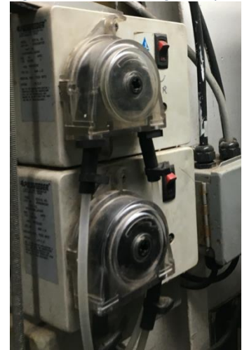
Figure 7 Chlorine Dosage Pumps
